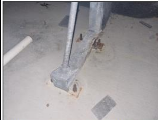
Photo 4 – Corrosion to base plates and bolted connections
