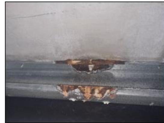
Photo 3 – Corrosion to 'Rondo' channel sections
